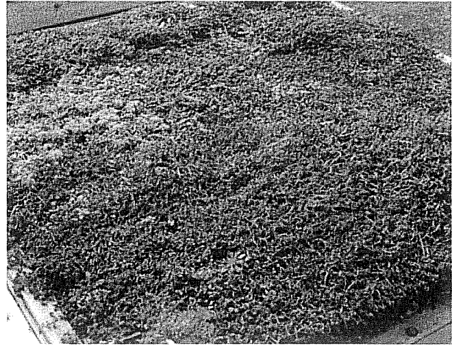
Plant coverage of the 4-inch vegetative system on Feb. 6, 2009. This photo shows full plant coverage of the surface.
